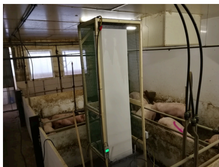
Figure 1: Practical trial for continuous adsorption of ammonia using innovative adsorber textiles at the Schulze Esking pig fattening farm, Billerbeck.
